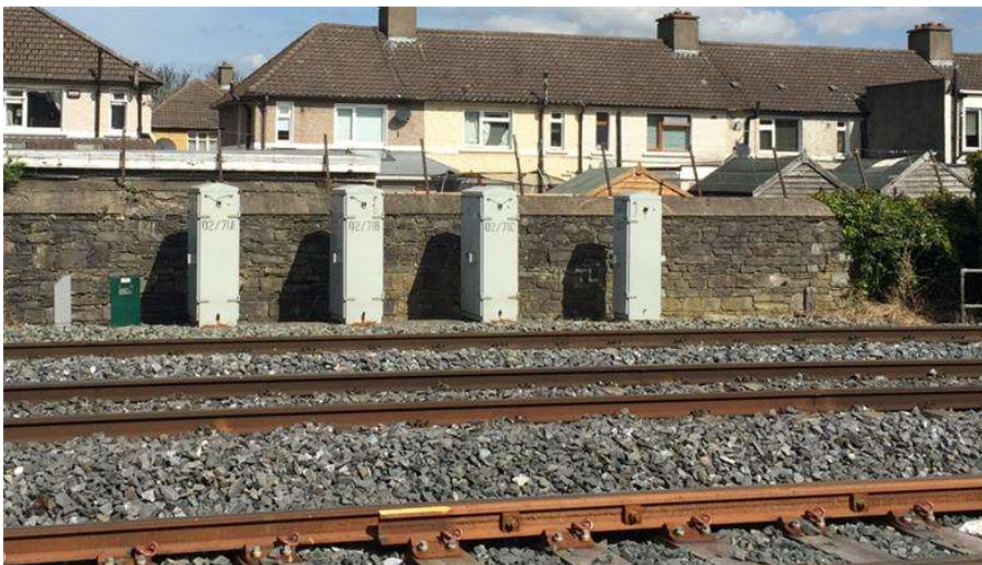
Figure 3-2 Examples of typical Object Controller Cabinet (OBJ) and Location Case
