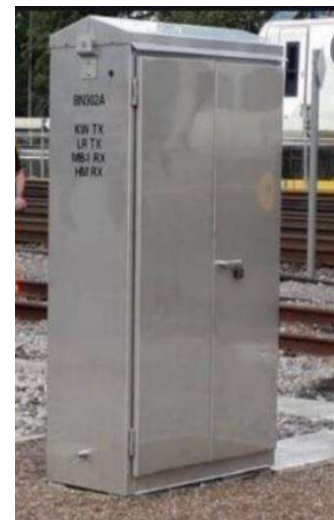
Figure 3-2 Examples of typical Object Controller Cabinet (OBJ) and Location Case
